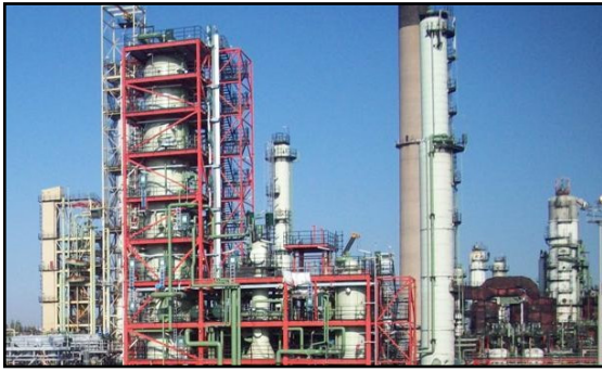
Biomass thermochemical processing unit at Porvoo (Finland)
