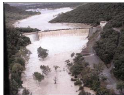
La Rouvière flood retarding dam during the flood of 9 September 2002 that was higher than its safety project flood. Source: AIGREF no. 19
