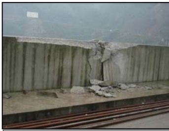
Cracks after an earthquake in China, May 2008 - Source : Bernard Goguel
